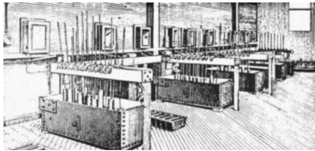
Şekil 2.3 İlk Charles Martin Hall hücreleri (Pittsburgh Reduction Company, 1888) (Yalvaç, 2003)
