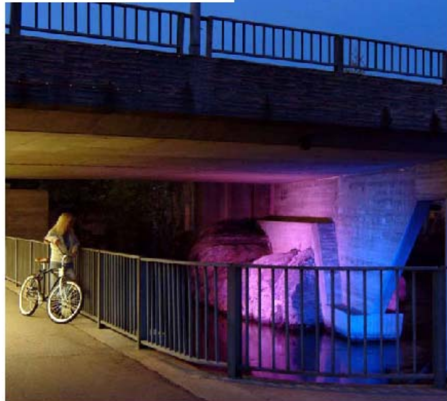
Location: Municipal Administration, Oak, Norway / Architect: Steinhilber / Lighting Designer: Jørge Oskalun
