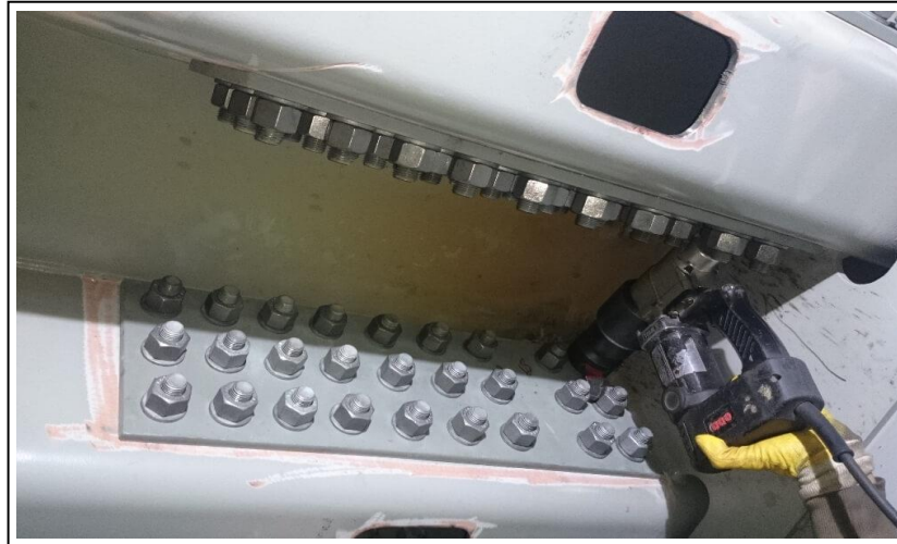
Figure 4.1 Bolted steel plates method [47]
