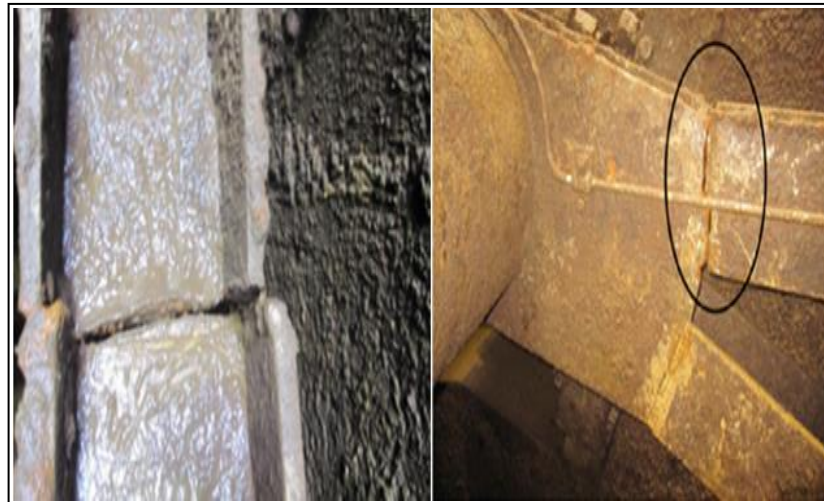
Figure 2.12 CFRP applied on struts of the valve [93]
