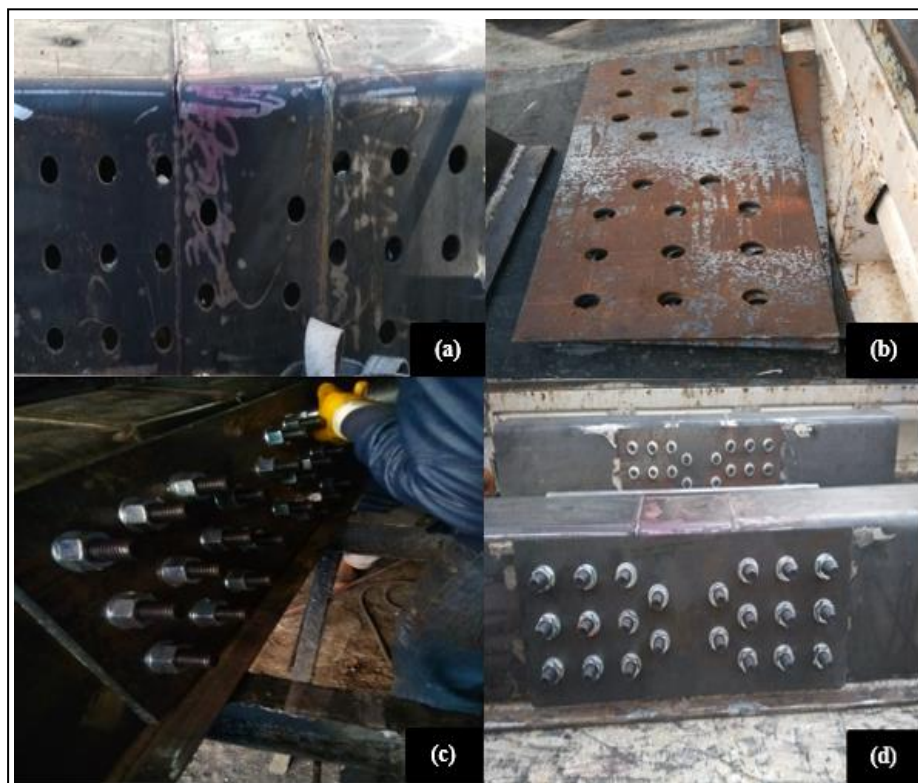
Figure 4.5 (a) Drilling the holes on the damaged ribs wall, (b) drilling the holes on the adding steel plates, (c) fastened the bolts, and (d) bolted steel plates to the damaged ribs wall
