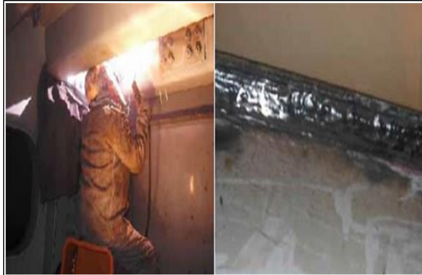
Figure 2.9 Welding treatment for a rib-deck crack, hanshin expressway [75]
