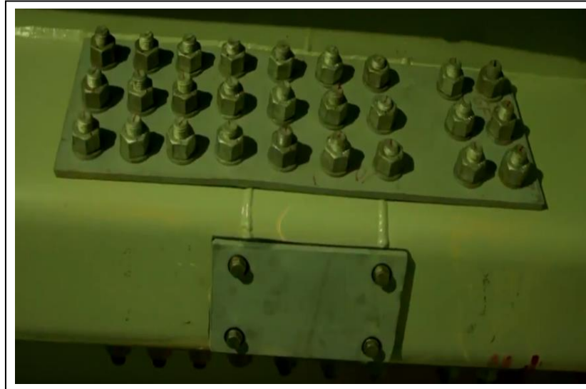
Figure 1.2 Faith sultan mehmet (FSM) bridge orthotropic crack repairs[47]
