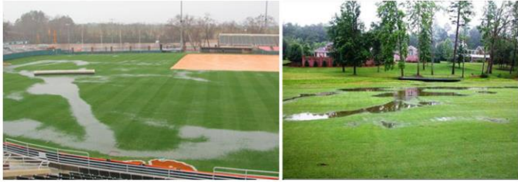
Figure 2.8 Insufficient Surface Drainage of Football Fields and Golf Greens (McCarty et al., 2016).
