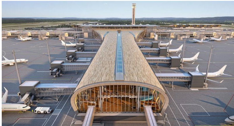
Şekil 3.43 Oslo Airport, Terminal 2 [159]
