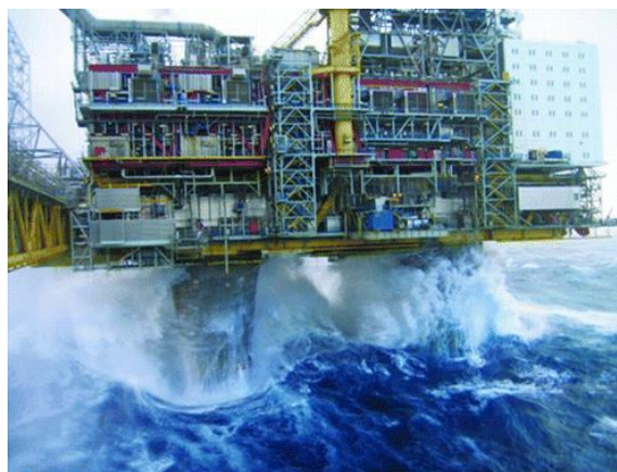
Figure 1.2 Slamming on offshore structure [2]
