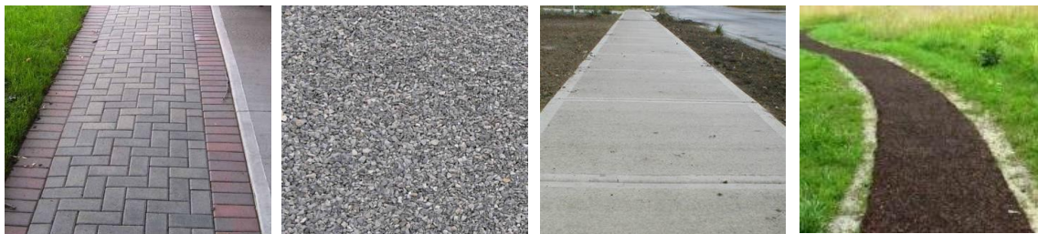
Figure 3.18 Recommended types of pathways surface, such as: "Brick; Finely Ground Stone; Brushed Concrete; and Rubber" [67].
