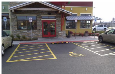
Figure 3.34 Accessible Parking with Wheel-Stop (Type A Spaces) [66].
