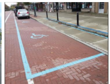
Figure 3.35 Accessible on-street parallel parking space "e.g. in the town center" [73], [66].
