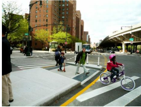
Figure 3.38 Pedestrian safety islands, New York City, USA [106].
