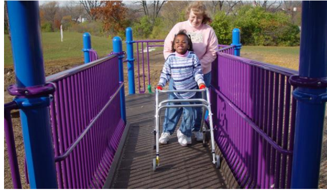
Figure 3.4 "Participation in Society": The route on the elevated composite structure is wide enough to accommodate a child using a walker [37].
