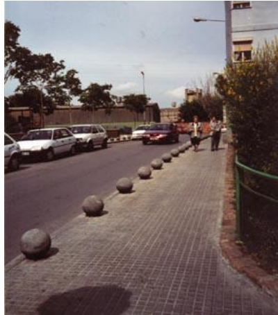
Figure 3.29 The balls clearly demarcate the boundary between vehicles and pedestrians but could also pose a trip hazard [75].
