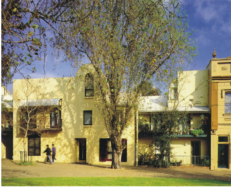
Şekil 4.26 Forbes Street Housing, Sydney, Avustralya, Cox Architects.
