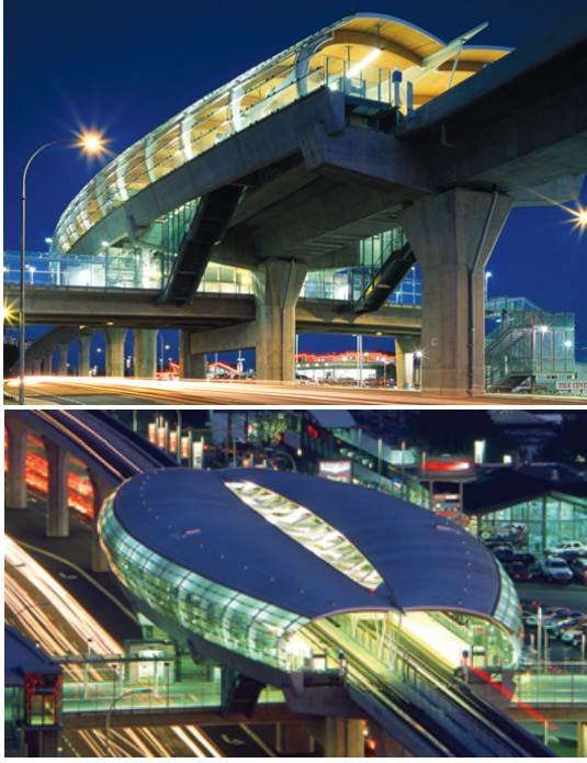
Çizelge 5.9 Brentwood Skytrain Station, Vancouver, Kanada [119], [120].
