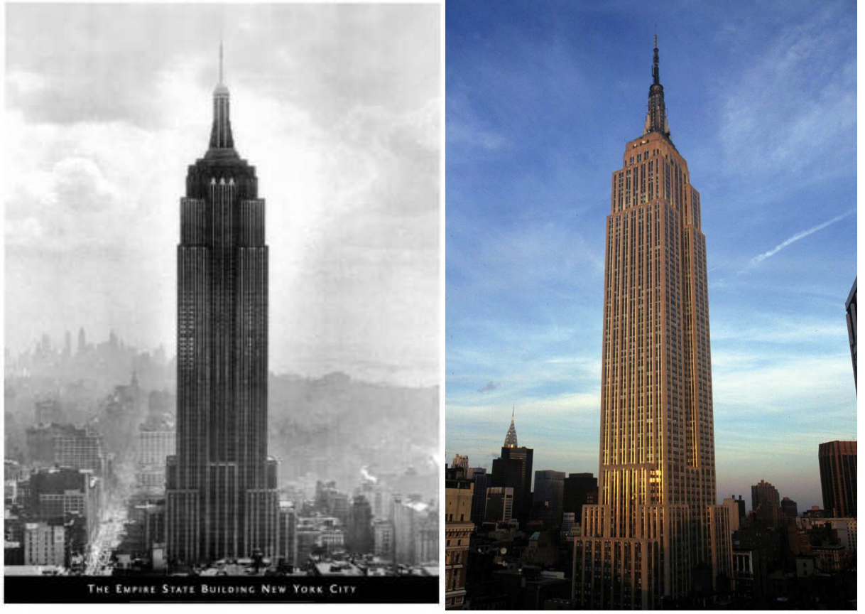
Şekil 4.19 Empire State Building.
