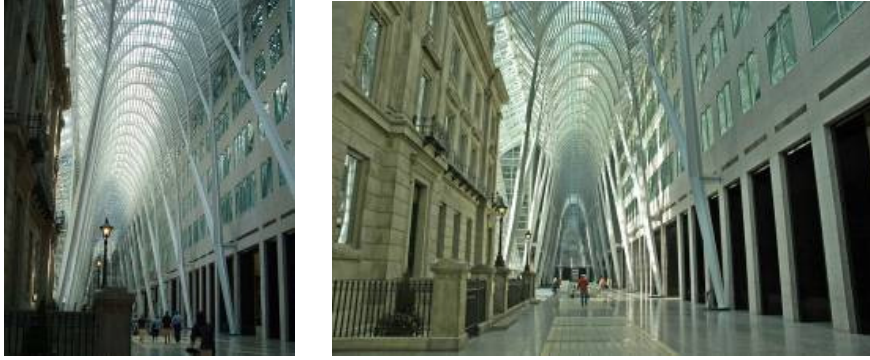
Şekil 4.2 BCE Place, Toronto, 1987, Santiago Calatrava [27-28].
