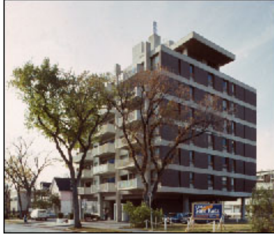
Şekil 2.25 Grosvenor House, Winnipeg, Kanada [11]
