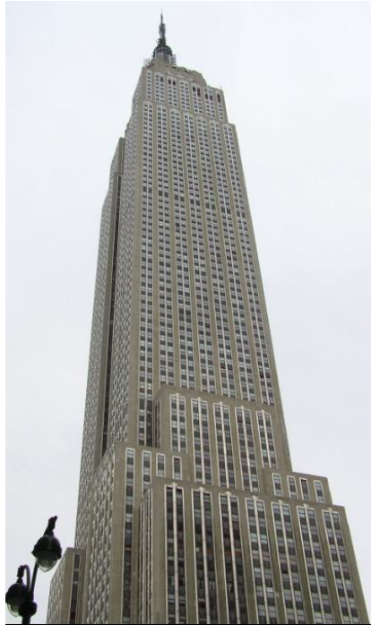
Şekil 2.7 Empire State Building
