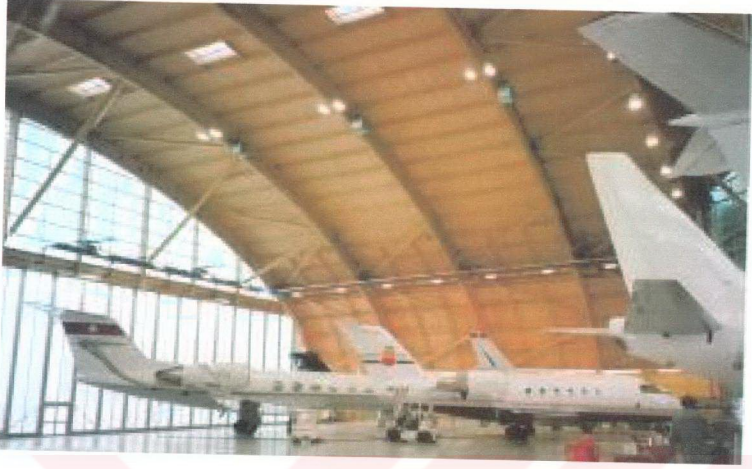
BÂLE AIRPORT BOEING 747 Hangar açıklık 82 metre (Mathis Company)
