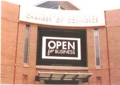
Şekil 3.75 Greater Little Rock Chamber Ctr., Little Rock, Arkansas
