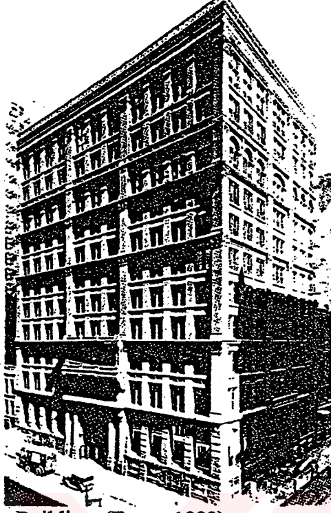
Şekil 3.3 Home Insurance Building (Ersoy, 1993)
